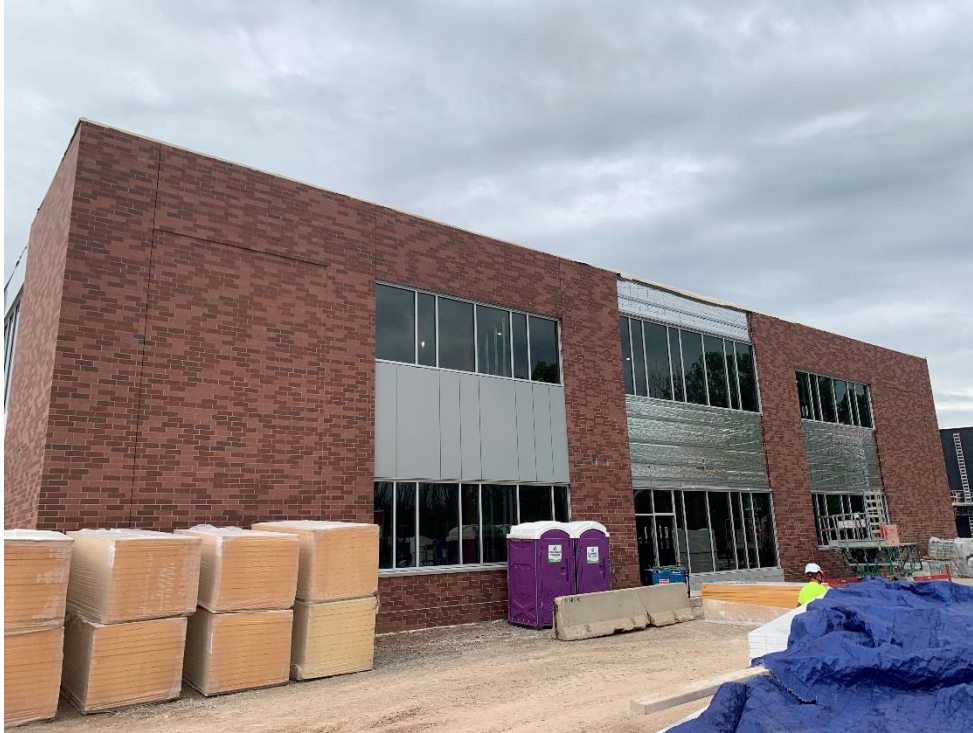
8. Area 5 – Metal panel girt system and storefront glazing installation in progress.
