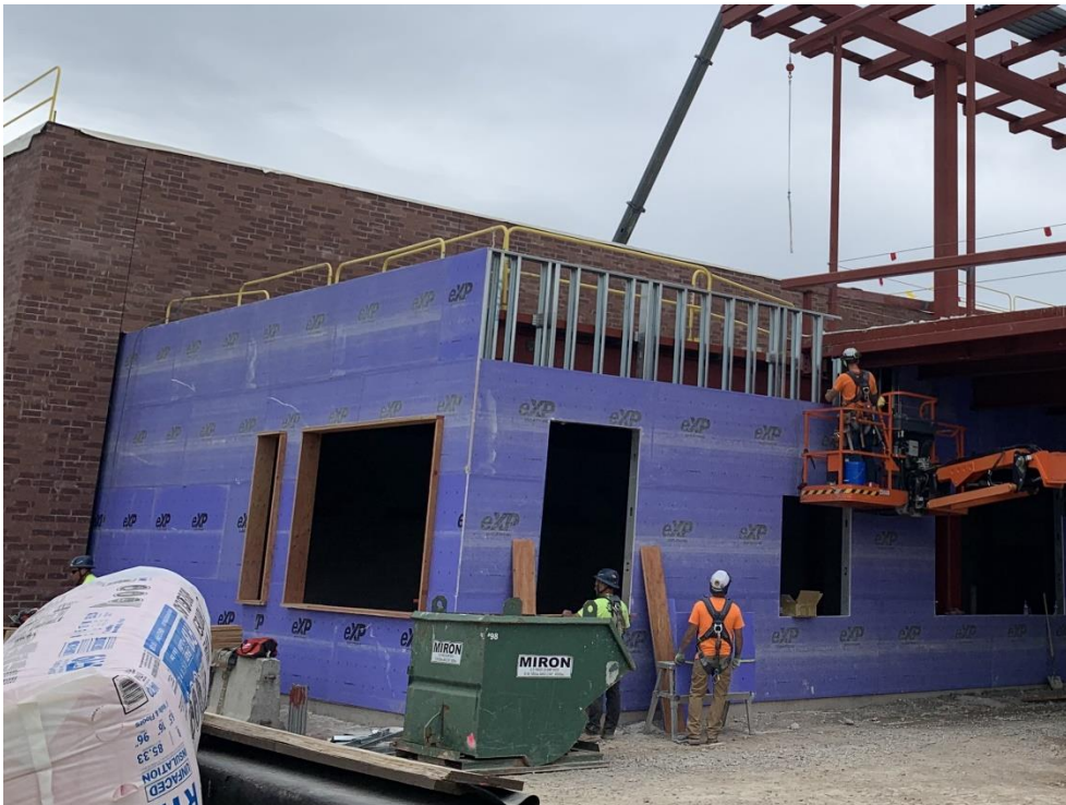
18. Area 1A – Exterior metal stud framing, sheathing, and window blocking installation in progress.
