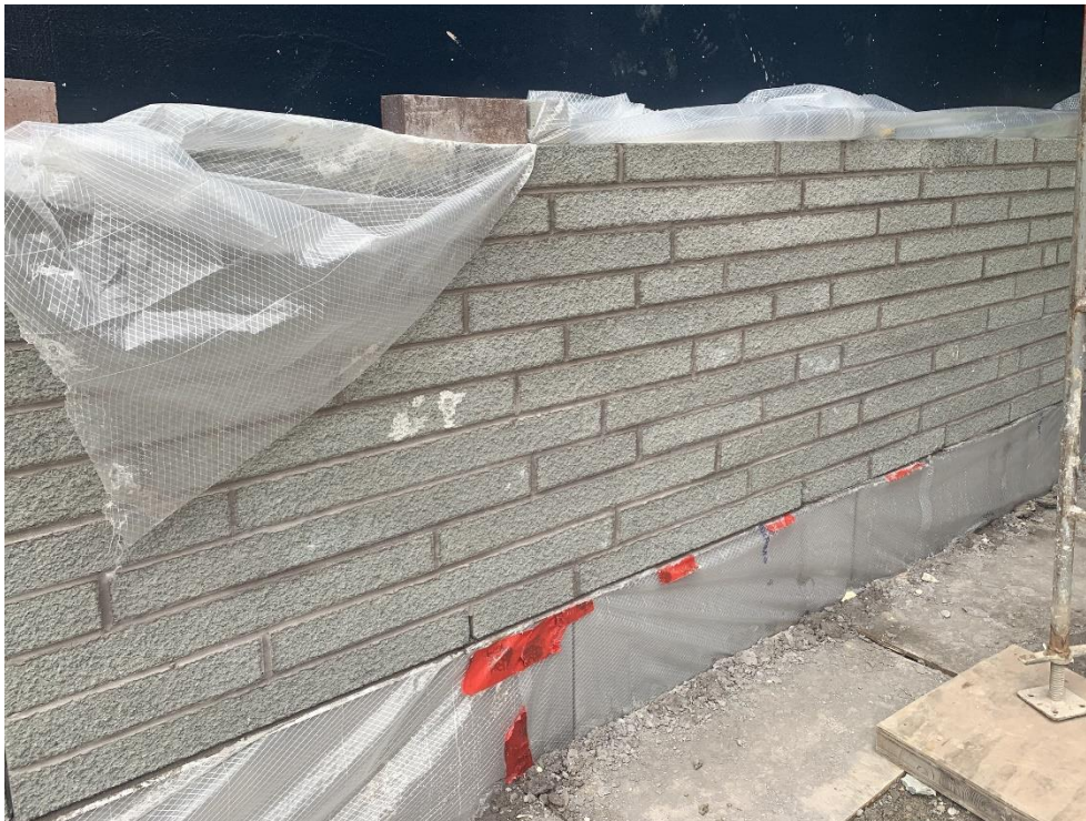
10. Area 5 – FB-2 random bond pattern installation in progress.
