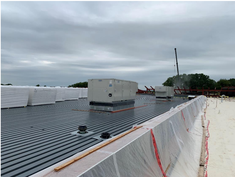
20. Area 6 – RTU and roof drain installation in progress.
