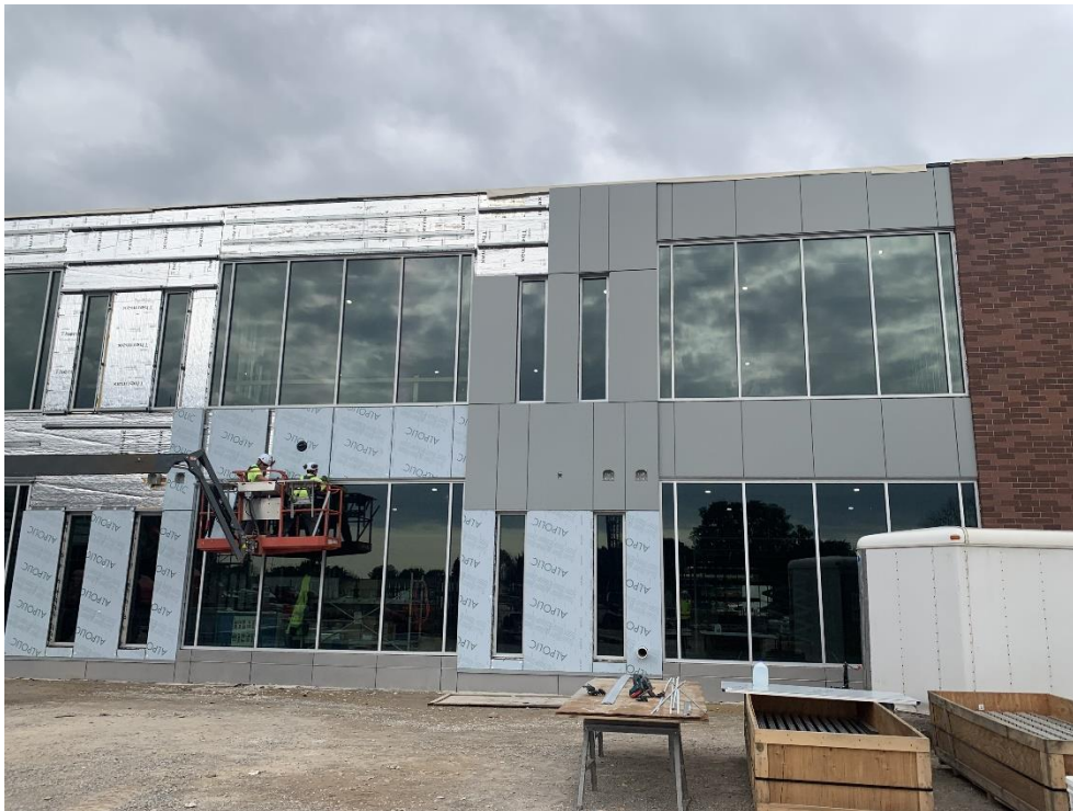
6. Area 5 – Composite metal panel and storefront glazing installation in progress.
