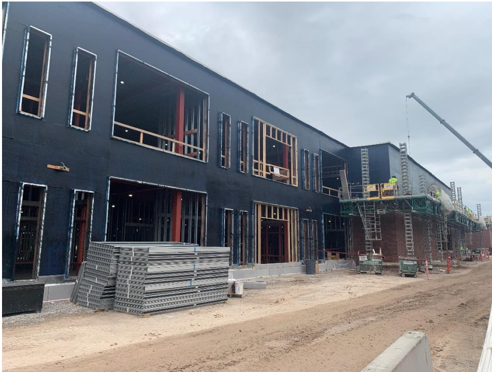
14. Area 3 – Exterior cast stone and window/door weather proofing membrane installation in progress.
