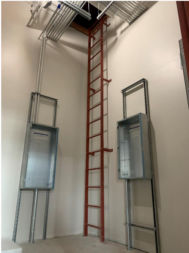
34. Area 5 – roof ladder and hatch. Electrical conduit installation in progress.
