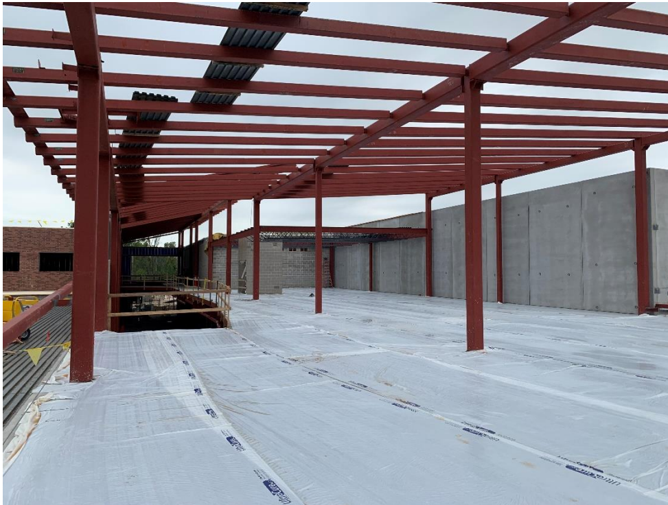
42. Area 1A – prep for slab on grade pour in progress.
