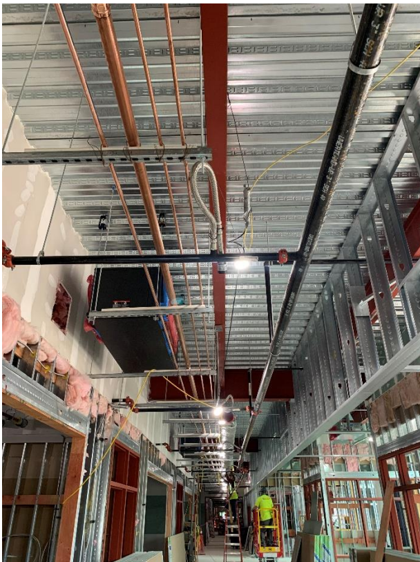
24. Area 6 – Above ceiling plumbing, fire protection piping, and geothermal pipes & heat pump installation in progress.
