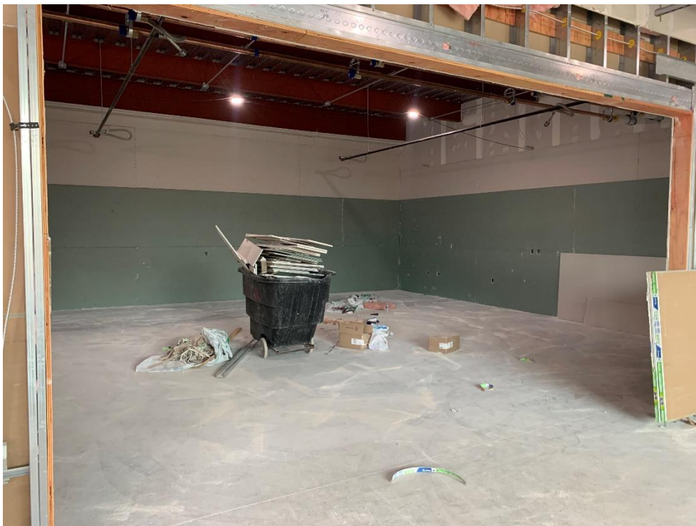
26. Area 6 – gyp board installation in progress.
