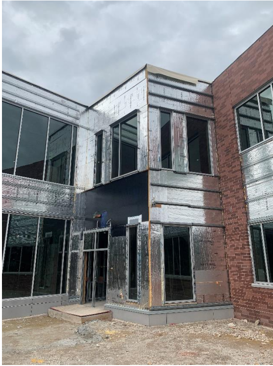
6. Area 5 – Composite metal panel and storefront glazing installation in progress.
