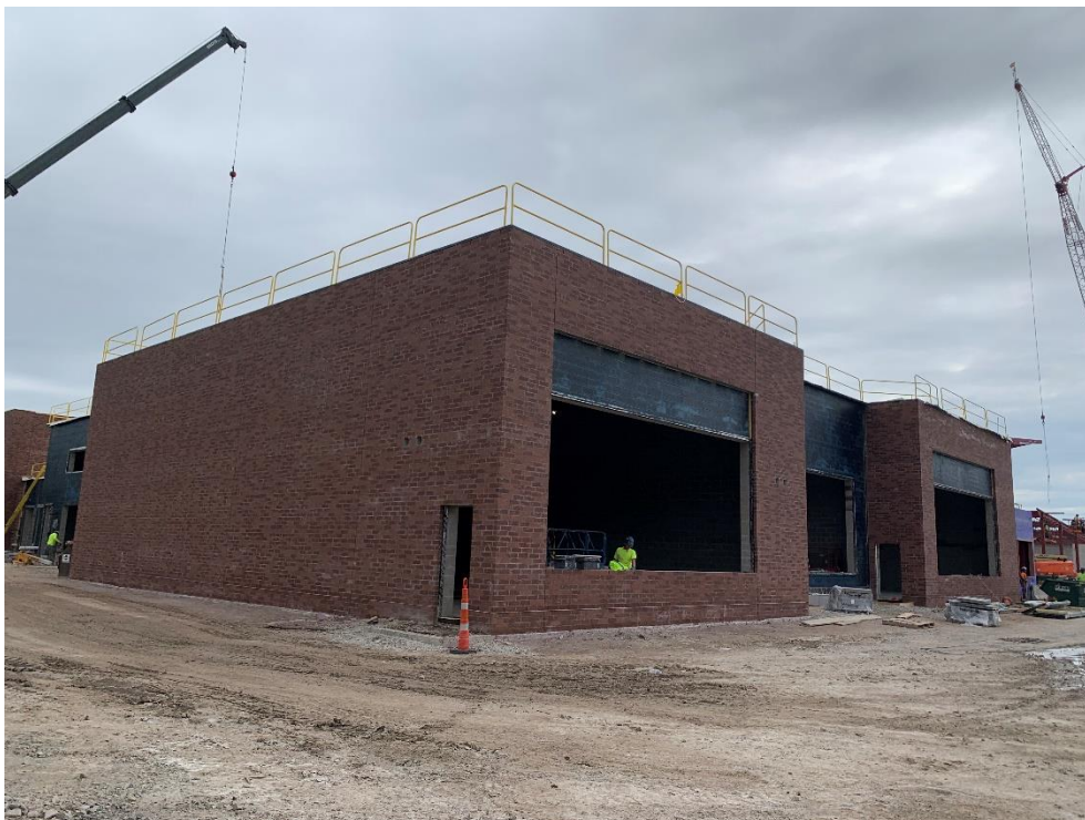
16. Area 2A – Exterior face brick veneer installed
