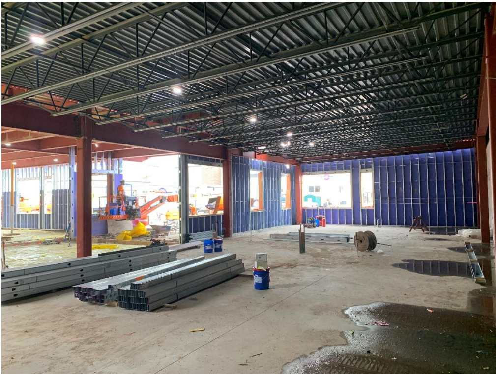
44. Area 1A – Interior metal stud framing in progress.
