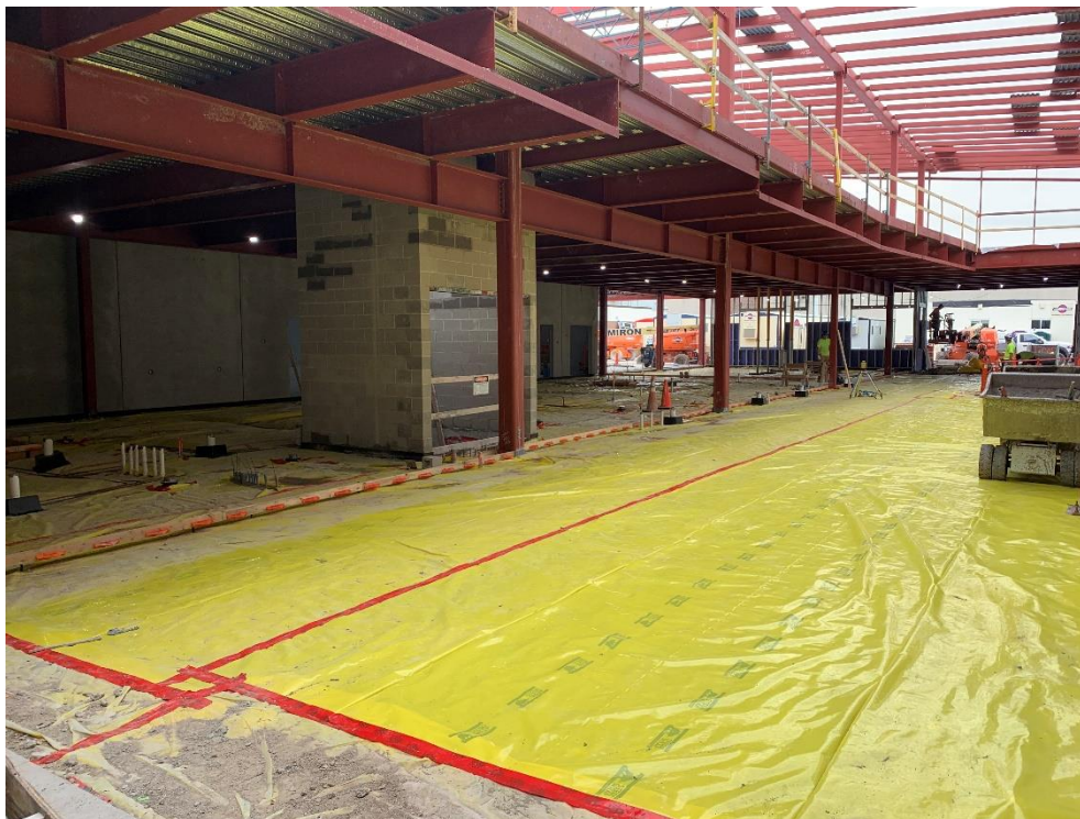
42. Area 1A – prep for slab on grade pour in progress.
