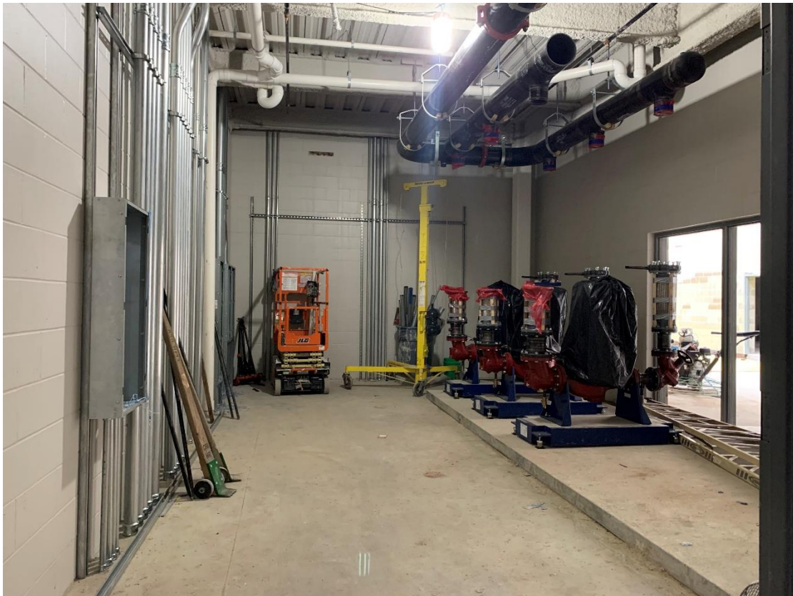
30. Area 6 – First floor pump room geothermal pumps, piping, and electrical conduit installation in progress.
