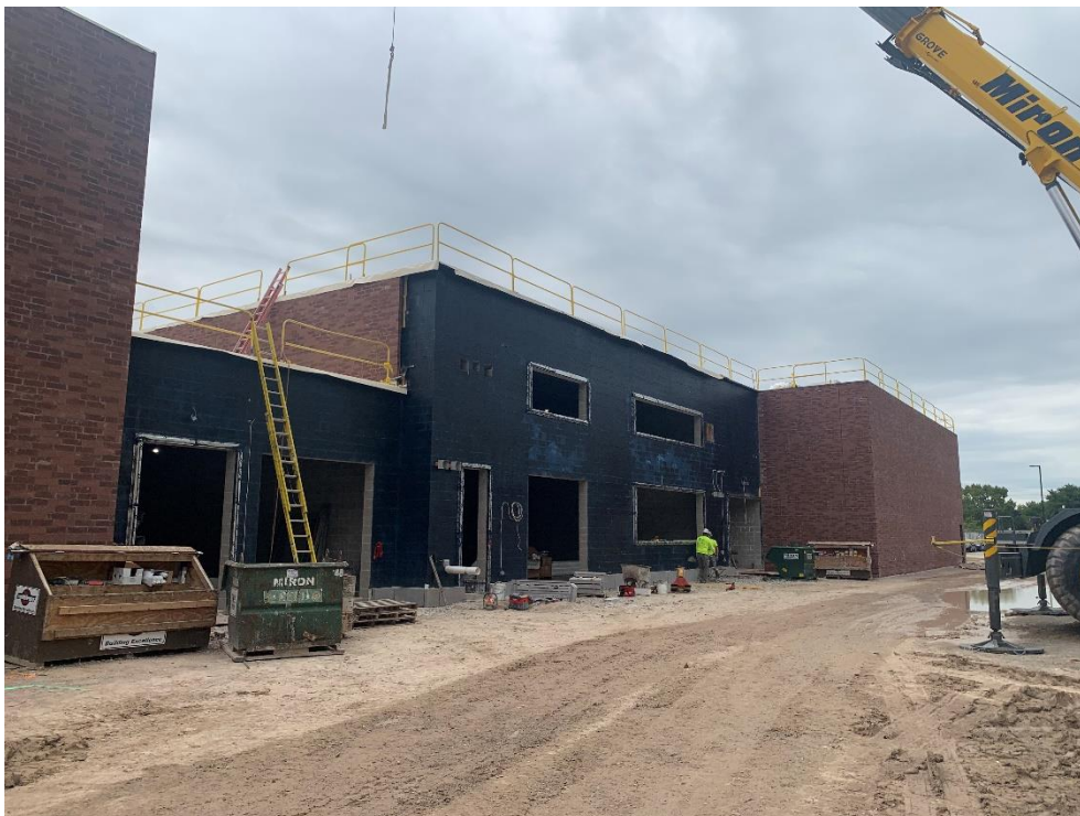
14. Area 3 – Exterior cast stone and window/door weather proofing membrane installation in progress.
