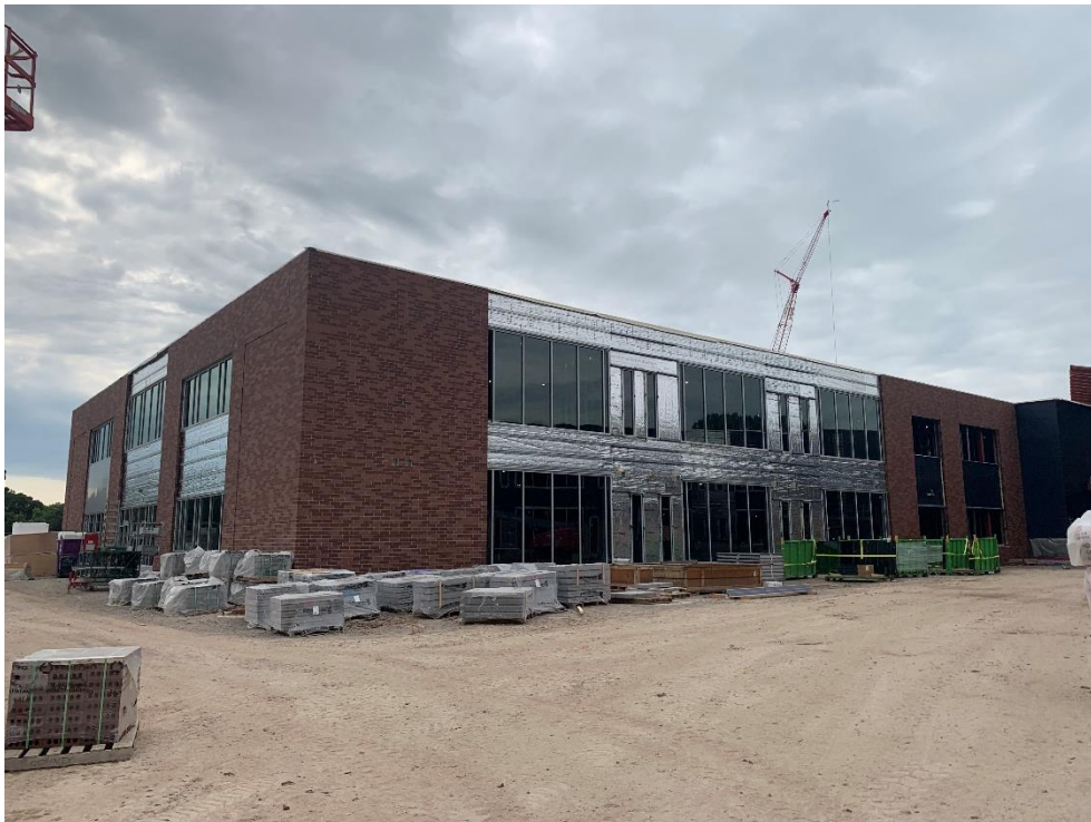
8. Area 5 – Metal panel girt system and storefront glazing installation in progress.
