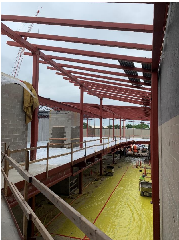
40. Area 1B – Roof decking installation in progress.
